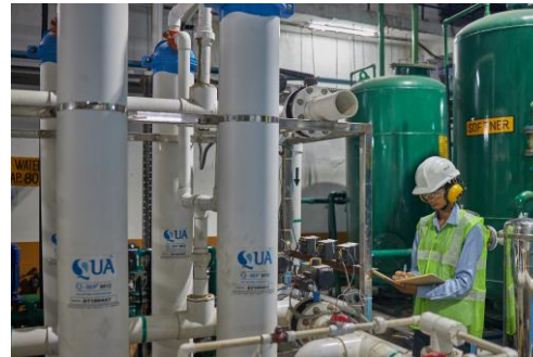
STP Plant with Ultra-filtration
